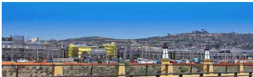
Under construction - 580,000 sq. ft. Outlets at San Clemente
